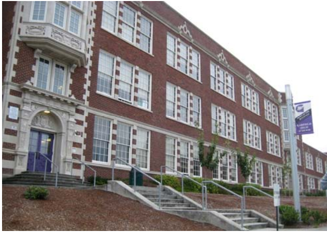
Exterior of school
