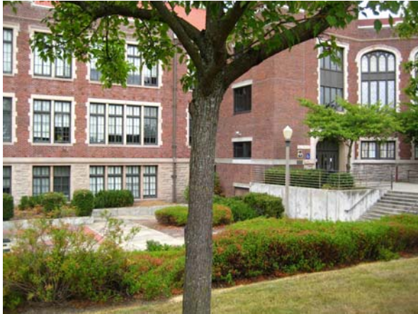
Exterior of school
