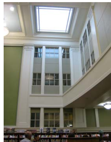
Skylights for more light- 2nd & 3rd story rooms gain access to the skylights
