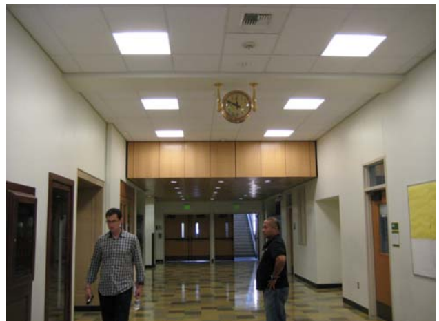
Soffit in hallway for additional MEP equip
