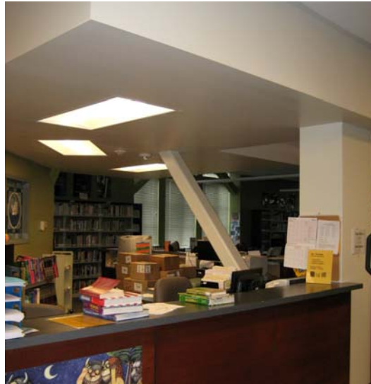
Library with new seismic bracing
