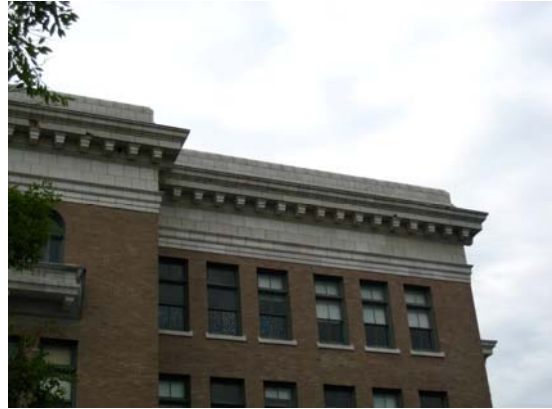
Corbels that had fallen off were replaced/repared.
