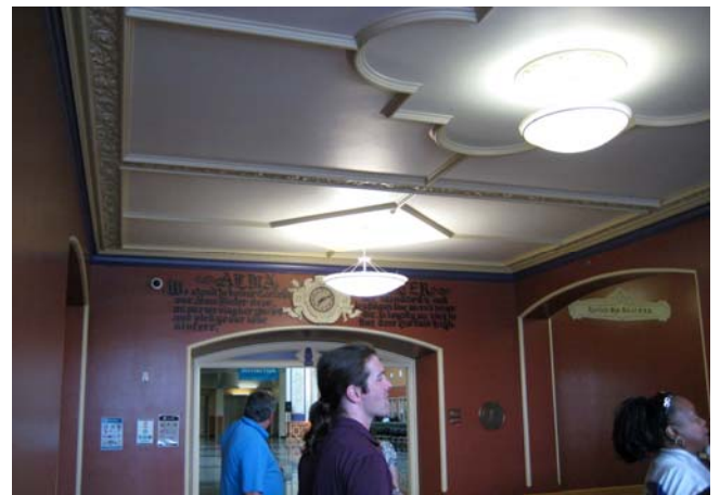
Entry lobby. Restored details.
