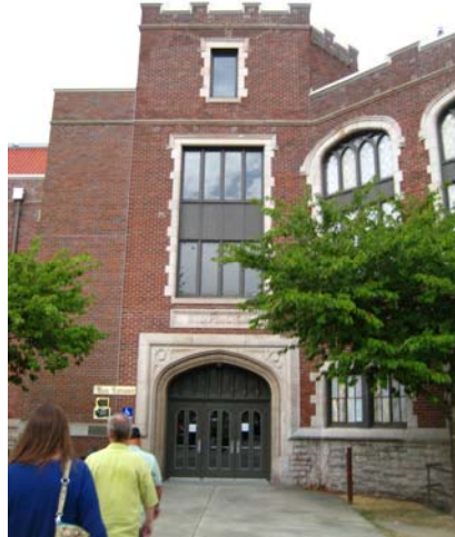
Main entrance (not well defined)
