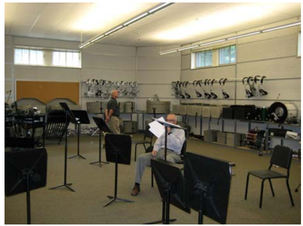
Music room (practice rooms used for storage)
